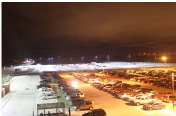
The LED lights (the white lights in background) used for the new parking lot in Winnipeg, Manitoba, Canada, make a measurable difference in lighting and energy savings, compared to the existing lights (orange-yellow lights in foreground). (Boeing photo)
