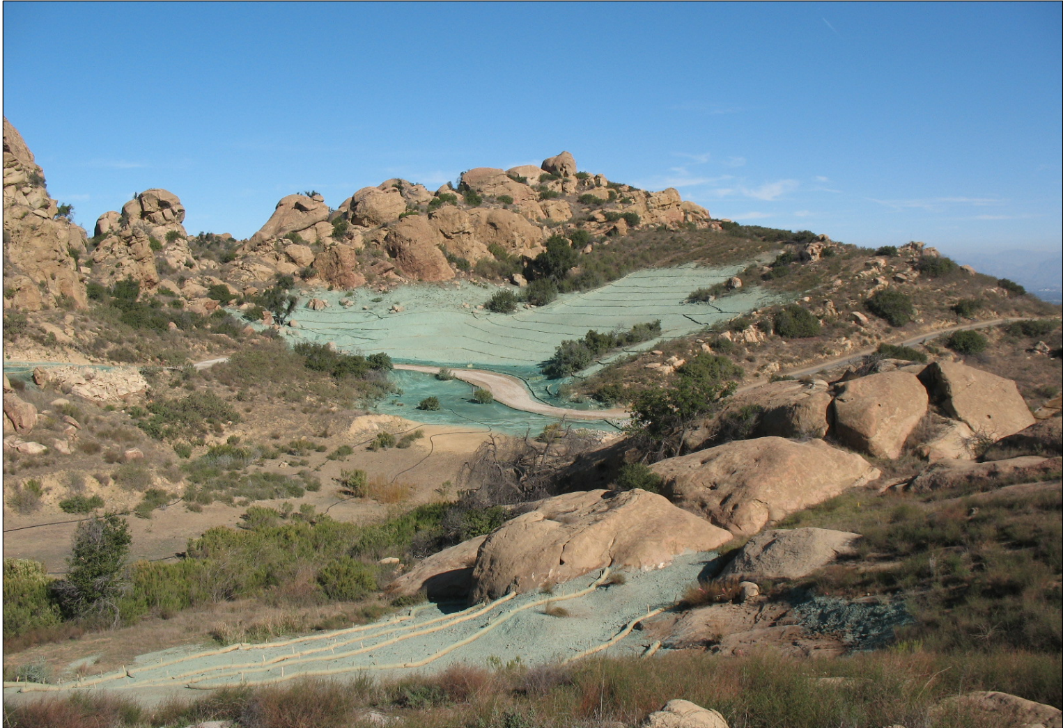
Outfall 008 ISRA Areas – Re-contoured and Hydroseeded
