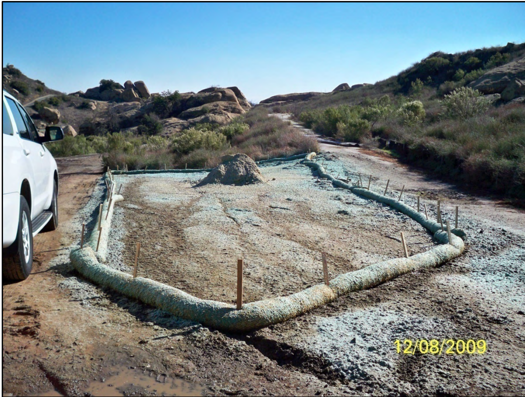
View looking southeast across completed HVS-4 ISRA Area, Happy Valley South, 12-8-09.
