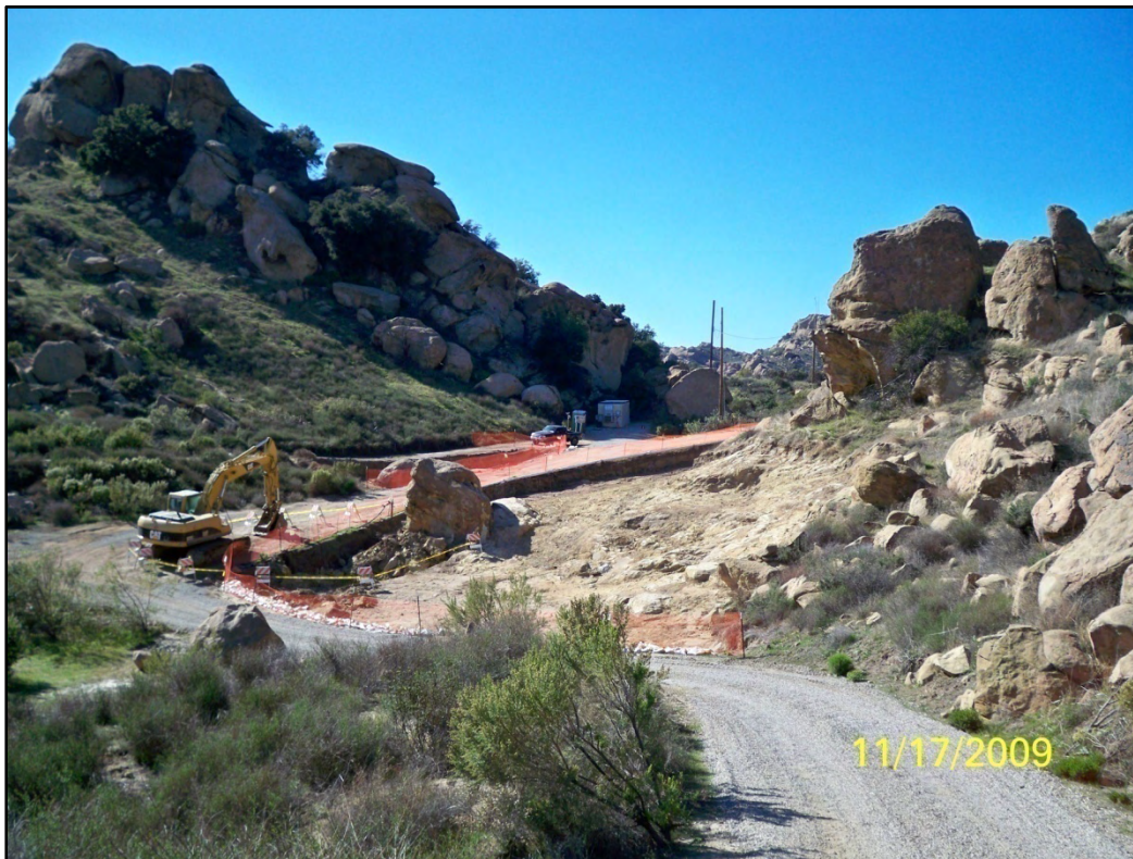
View looking west across post-excavation HVS-3 ISRA Area, Happy Valley South, 11-17-09.
