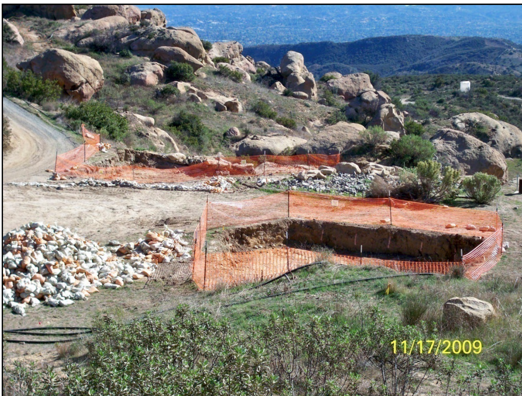
View looking southeast at post-excitation HVS-2B-1 ISRA Area (foreground), Happy Valley South, 11-17-09.
