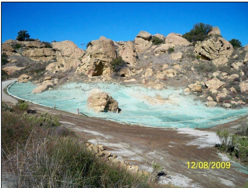
View looking north across completed HVS-3 ISRA Area, Happy Valley South, 12-8-09.
