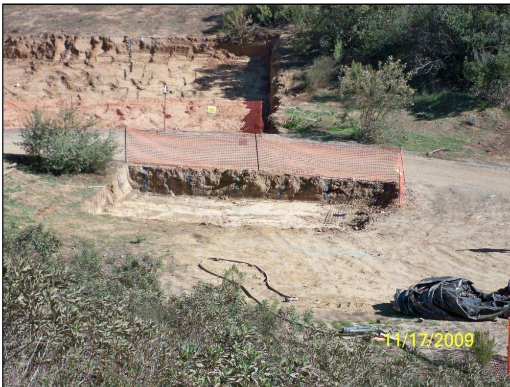
View looking east across post-excavation HVS-2D ISRA Area, Happy Valley South, 11-17-09.
