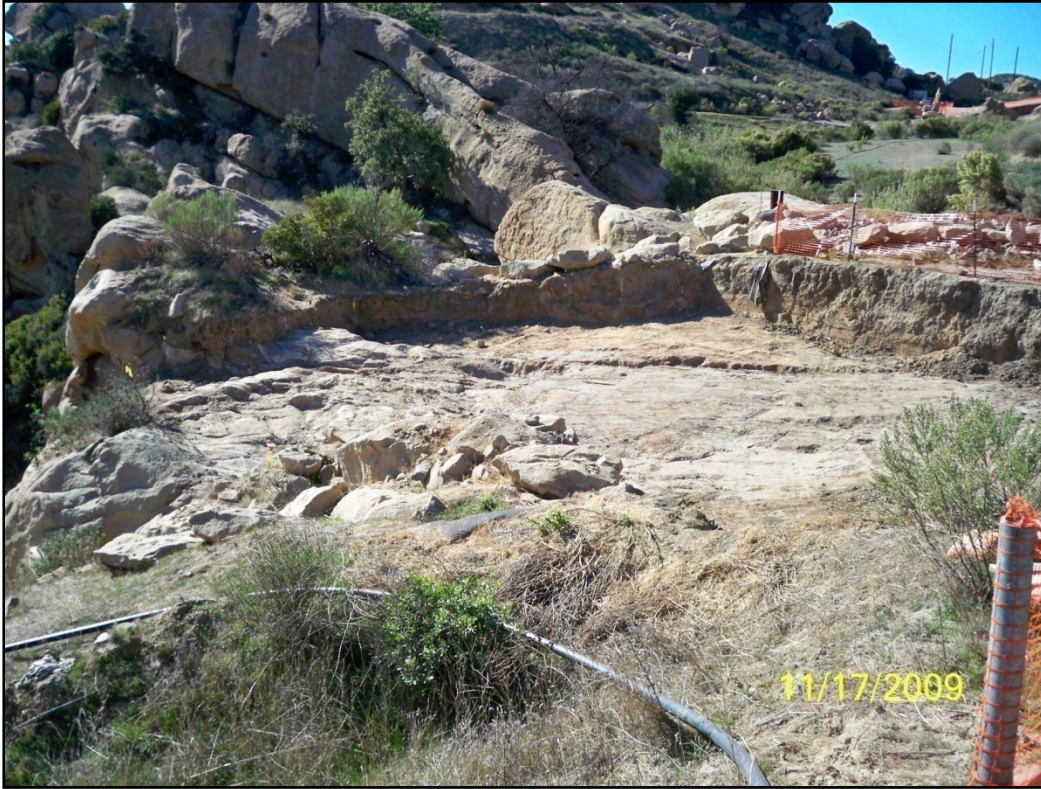
View looking west across post-excavation HVS-2B-2 ISRA Area, Happy Valley South, 11-17-09.
