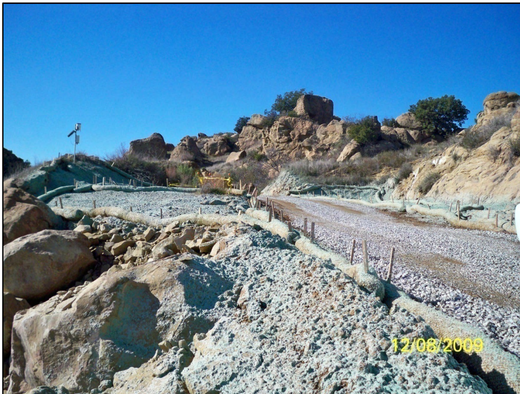
View looking west across restored HVS-2C ISRA Area, Happy Valley South, 12-8-09.
