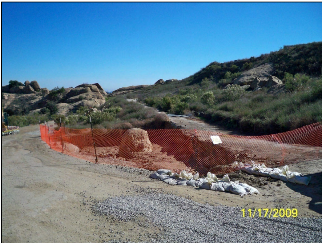
View looking southeast across post-excavation HVS-4 ISRA Area, Happy Valley South, 11-17-09.
