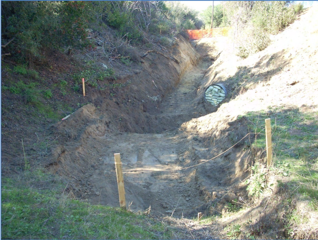
View looking northwest across post-excavation A2LF-3 ISRA Area, Outfall 009, 11-16-09.
