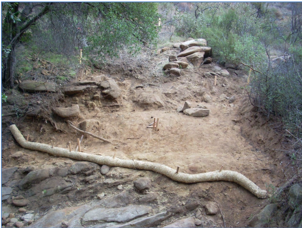
View looking northeast across post-excavation A2LF-1 ISRA Area, Outfall 009, 11-10-09.
