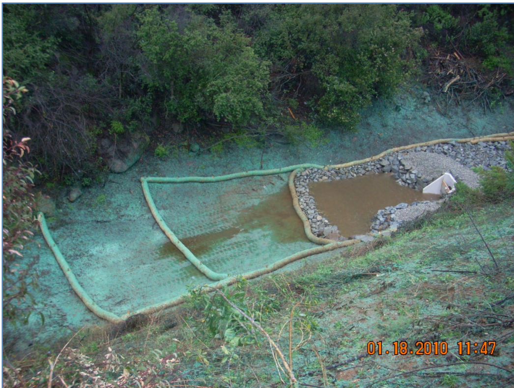
View looking south across completed A2LF-3 ISRA Area, Outfall 009, 1-18-10.
