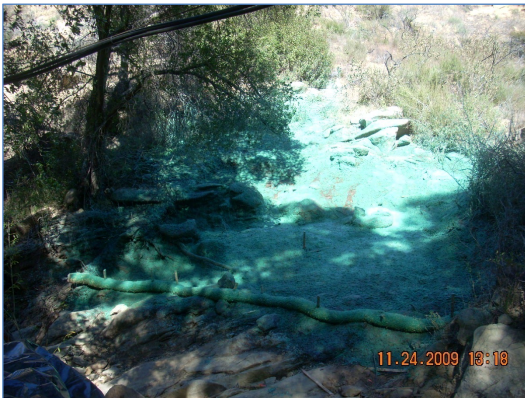
View looking northeast across completed A2LF-1 ISRA Area, Outfall 009, 11-24-09.
