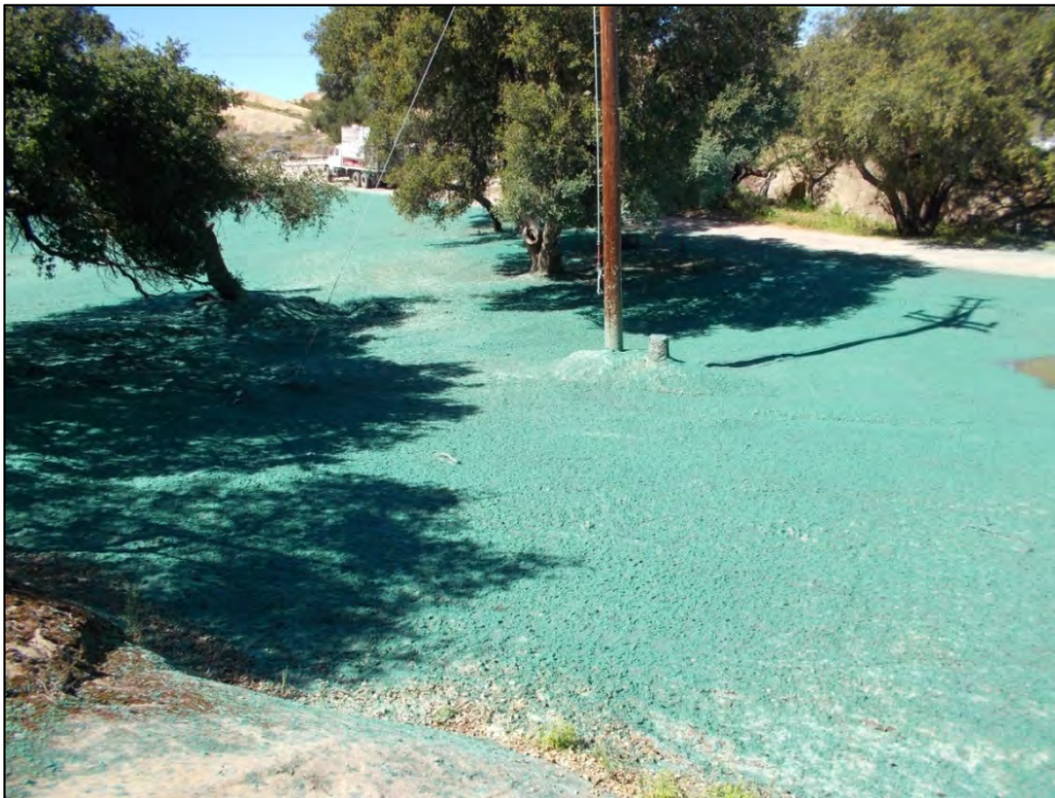
View of ISRA area AP/STP-1B (eastern portion) after hydroseed application (3/8/2013, looking northwest).
