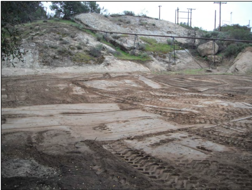
View of ISRA area AP/STP-1B during soil contouring of western portion prior to hydroseeding (3/5/2013, looking south-southwest).
