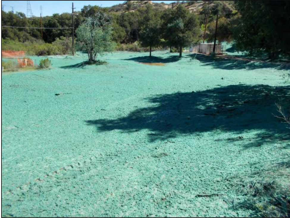
View of ISRA area AP/STP-1C-1 (western portion) after hydroseed application (3/8/2013, looking southeast).
