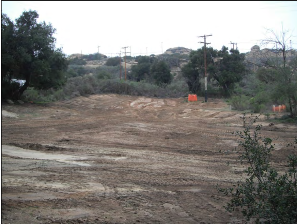
View of ISRA area AP/STP-1C-1 (western portion) after contouring (3/4/2013, looking northwest).
