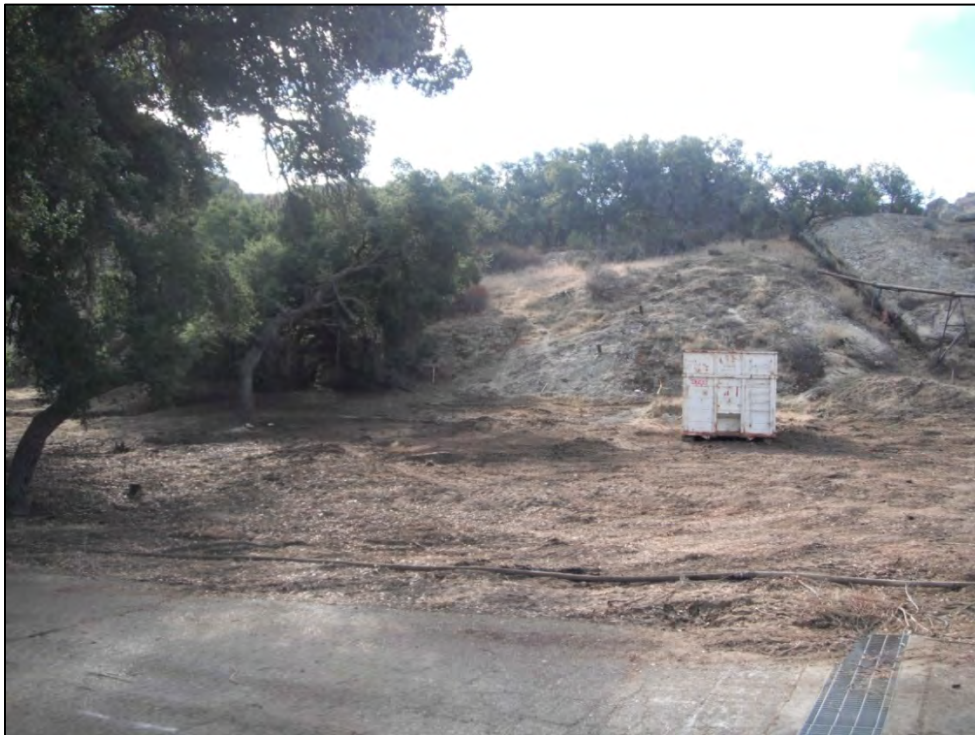
View of ISRA area AP/STP-1B prior to excavation (10/14/2011, looking south).
