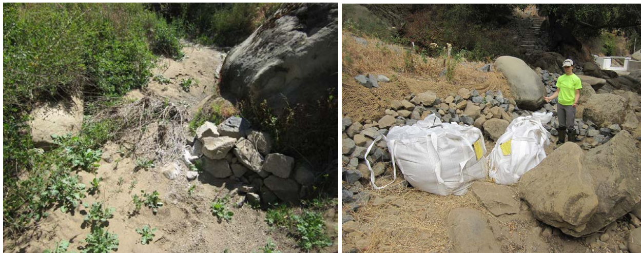
Figure 5. Northern Drainage Accumulated Sediment (left) and Sediment Collected in Super Sacks for Removal (right)
