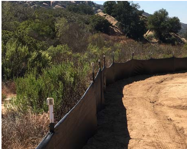
2017: Enhanced Erosion Controls in Former Shooting Range Area
