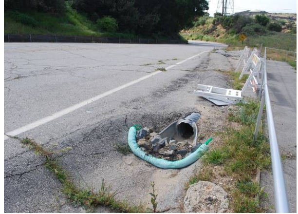
2017: Administration Area Inlet Filters (Weighted Wattle)
