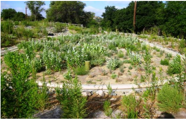
2013: Lower Parking Lot Sedimentation Basin and Biofilter
