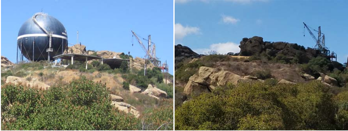
Figure 9. Hydrogen Gas Storage Area before (left) and after (right) Demolition
