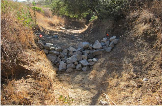
2012: Northern Drainage Restoration Measures
