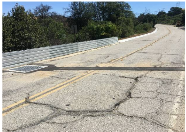
2017: Roadway Diversion to CM-3
