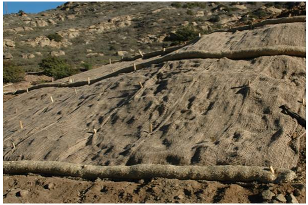
2013: Outfall 009 ISRA Excavations
