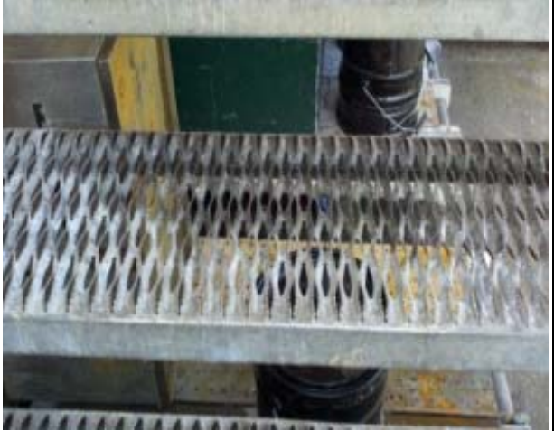
Stairs, galvanized; Everett
