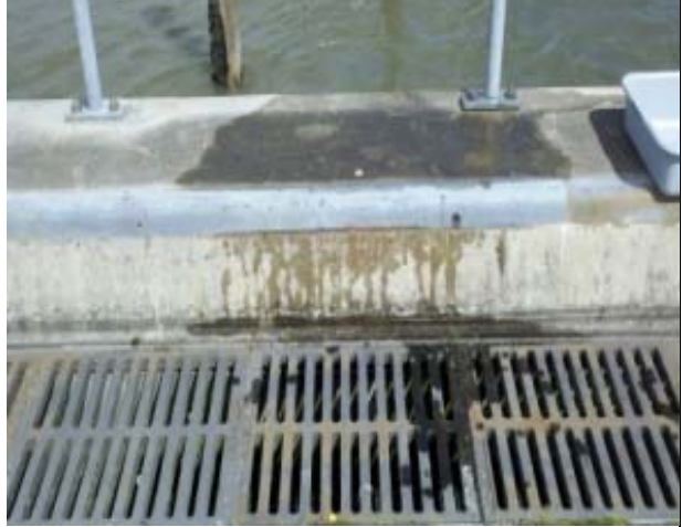
Sheath, over concrete barrier edge; Everett
