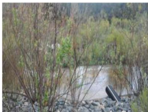
Figure 52. A photo of the biofilter on 3/13/2018
