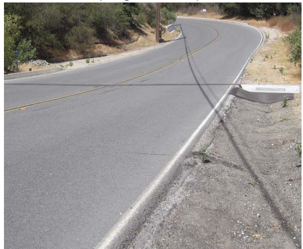
2017: Roadway Diversion to CM-1
