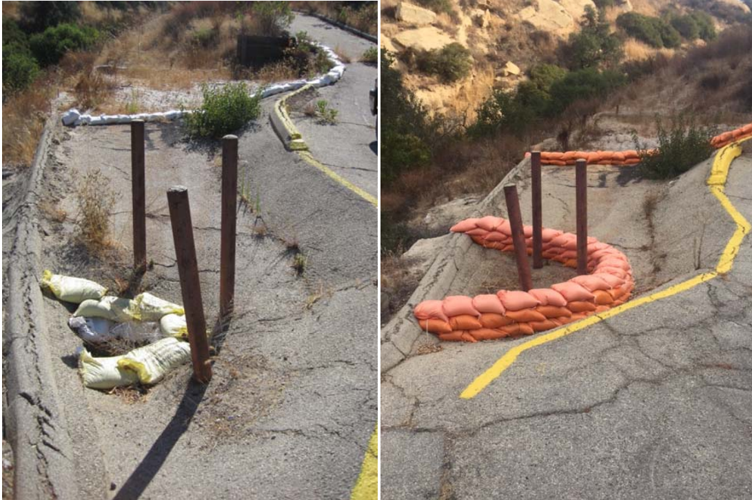
Figure 12. Well 13 Road Culvert Inlet before (left) and after (right) Improvement
