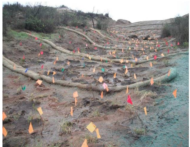
2010: Outfall 008 ISRA Excavations
