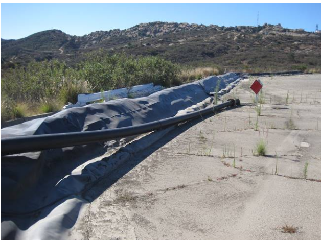
2011: Helipad Berms and Pumps
