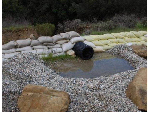
2013: LOX Sandbag Berms and Slope Drains
