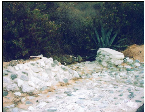
Grouted riprap; http://www.fs.fed.us/eng/pubs/html/wr_p/99771804/images/fig11.jpg
