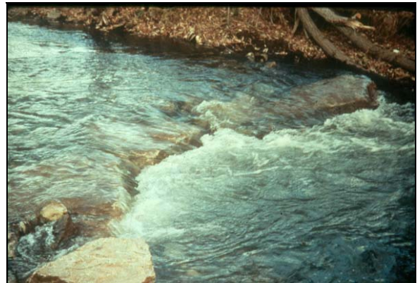
Riprap Check Structure photos from E-SenSS; Salix, 2004
