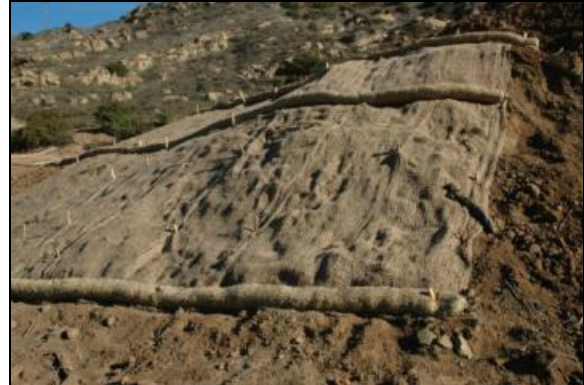
Erosion Control Blanket Placed at Boeing SSFL; Geosyntec, 2010
