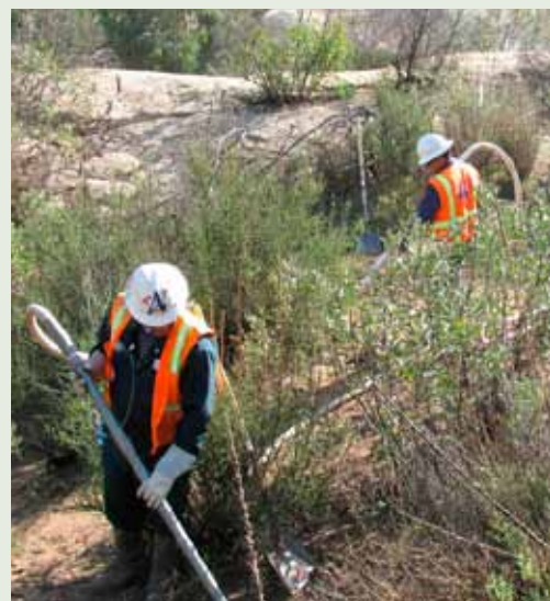
Workers use hand vacuums to remove lead shot from the rock outcrops on Sage Ranch.
