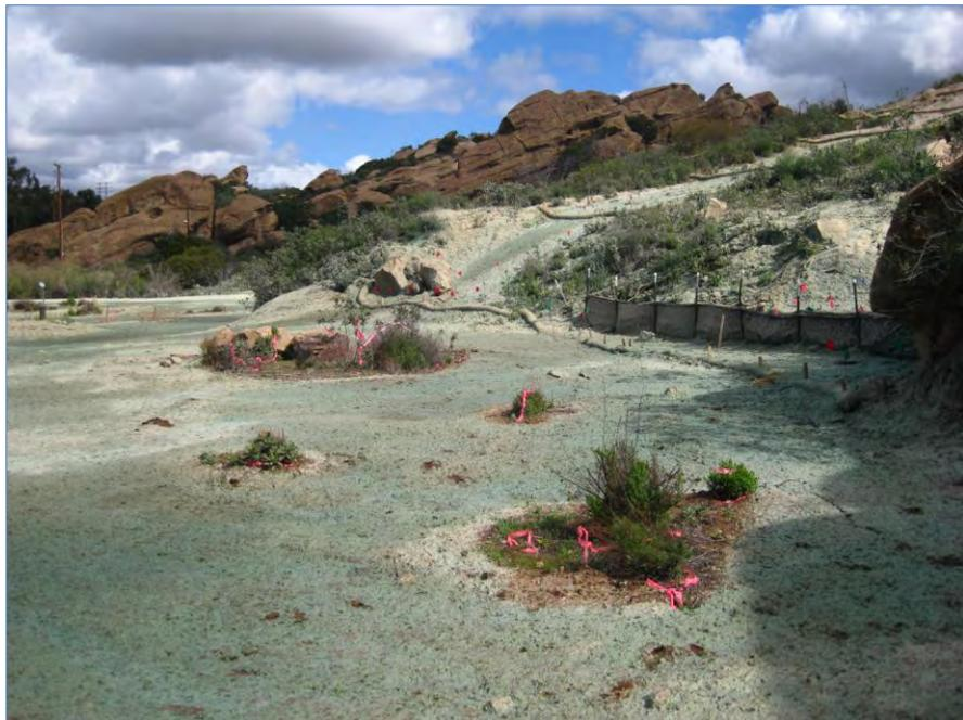
Figure 2. View of B1-1A subsequent to ISRA activities. Photograph is toward the north, taken on February 17, 2011. Site is hydroseeded, Santa Susana tarplants are present (marked by pink flagging) and BMPs are placed on hillside.
