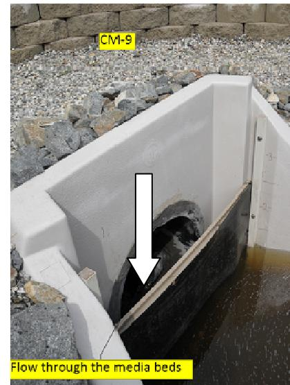
Figure 32. Filter media underdrain collection point
