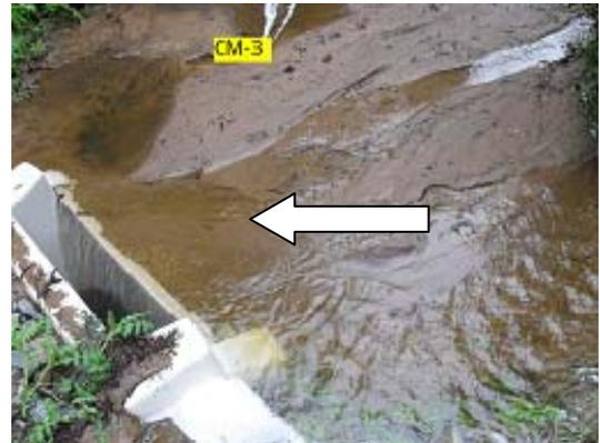
**Figure 11. Sediment accumulated behind weir boards at CM-3.**
