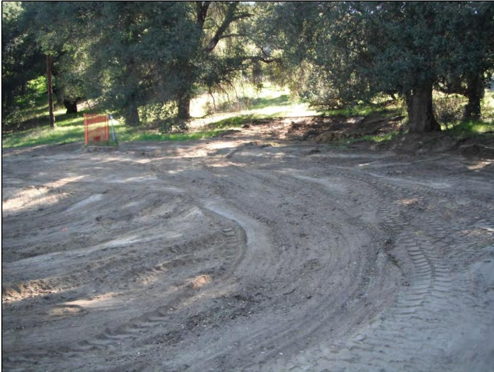
View of ISRA area AP/STP-1E-3 during soil contouring and prior to hydroseed application (2/28/2013, looking southeast).
