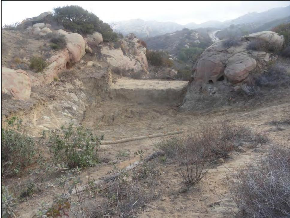
View of ISRA area ELV-1D excavation after contouring and installation of jute matting and fiber rolls (11/20/2013, looking east).
