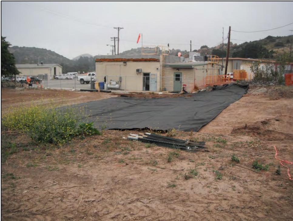
View of ISRA area IEL-2 during liner placement over gravel backfill (6/7/2011, looking east).
