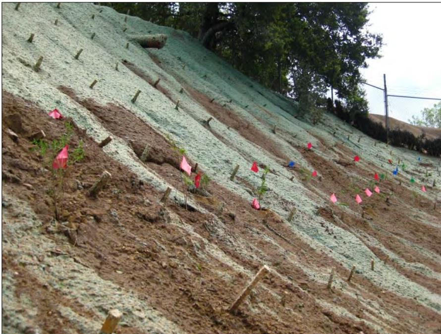
Figure B4. View of B1-2 planting area on March 21, 2011. Plantings were installed, and slope was covered in jute netting and hydroseeded.
