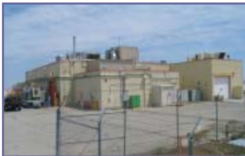
IMF at Edwards AFB, used for storing and processing ABL laser chemicals
