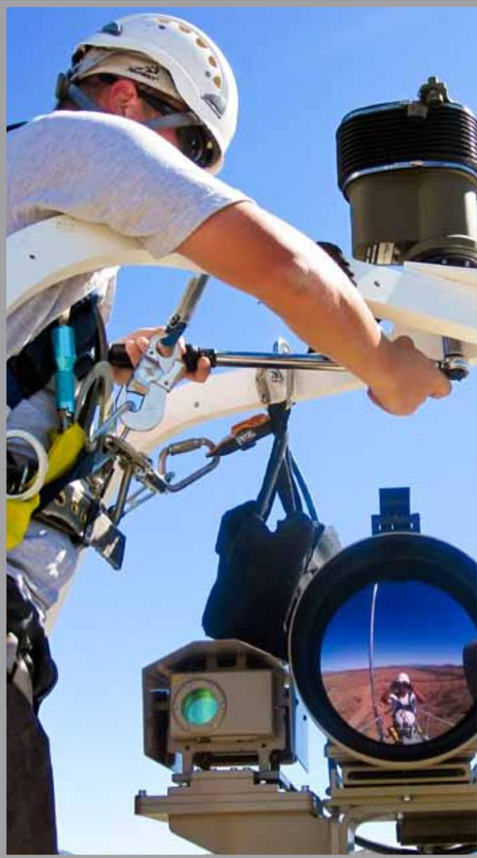
training, Peck can only access the top of the tower via a bucket lift but still dresses in a full harness, hooking to an anchor point on the bucket. Once he safely makes the transfer from the bucket and hooks his lanyard to the platform, he begins verifying that all the tower’s radio and sensor connections have been completed correctly by program subcontractors.
