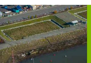
Left: At Plant 2 in Seattle, Washington, Boeing installed a biofiltration system to help improve the water quality of the neighboring Duwamish Waterway. The passive system treats an average of 84 million gallons (318 million liters) of stormwater annually. (Boeing photo)
