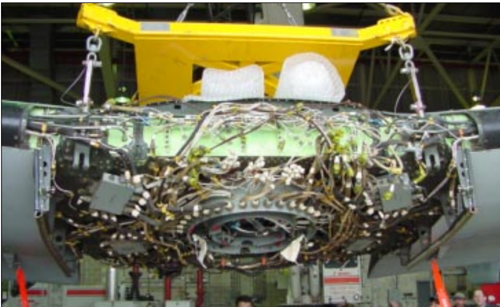
The Bell Boeing team completed the removal and delivery of the wing to Ft. Worth, Texas, within nine days, nearly three weeks ahead of the original time estimate.
