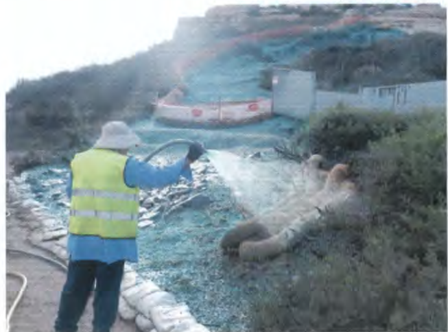
Applying hydroseed/mulch at B-1 access road.
