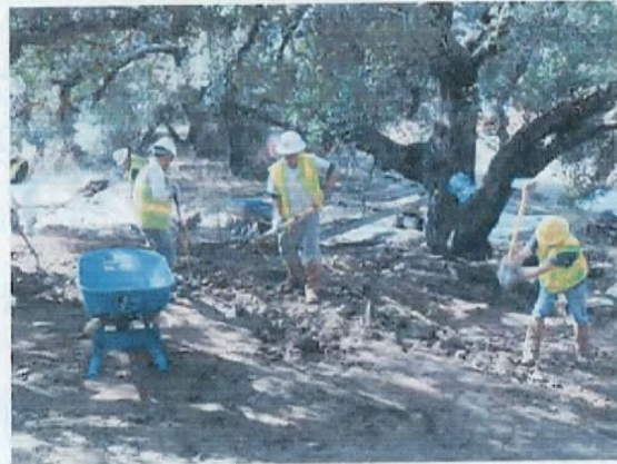
Excavating soil at AP/STP-1F using hand tools.
