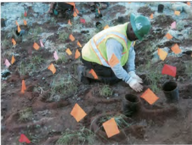
Installing plants at ISRA area CTLI-1B.
