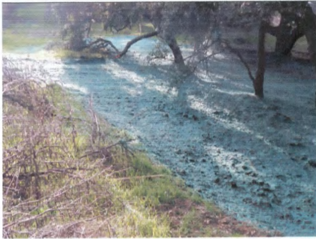
Re-contoured ISRA area AP/STP-1D, with hydroseed/mulch.
