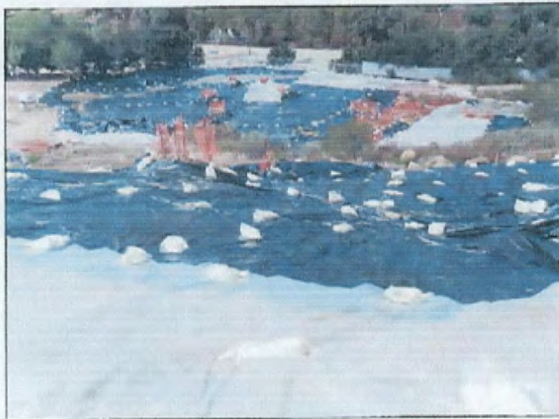
ISRA Areas B1-1D (foreground) and B1-2 (background) covered with plastic in preparation for rain event.
