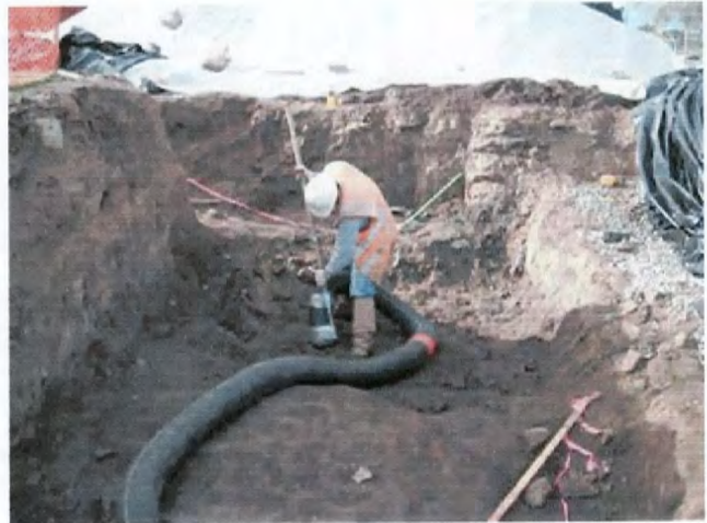
Additional excavation at ISRA area B1-2 with supervac.
