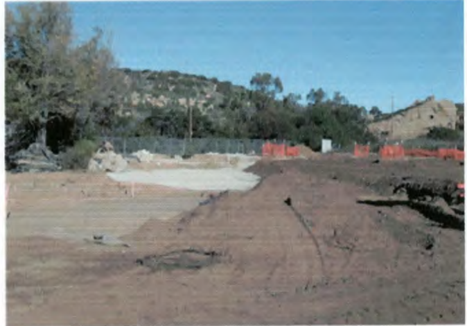
Backfilling and re-contouring completed portions of ISRA area B1-2.
