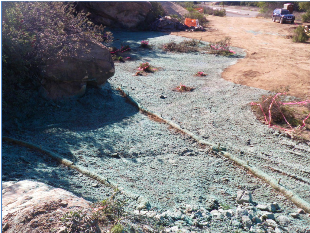
ISRA area B1-1A after restoration (11/16/2010, looking southwest). Blue-green hydroseed mulch is visible. Orange flagging tape identifies Santa Susana tar plants.
