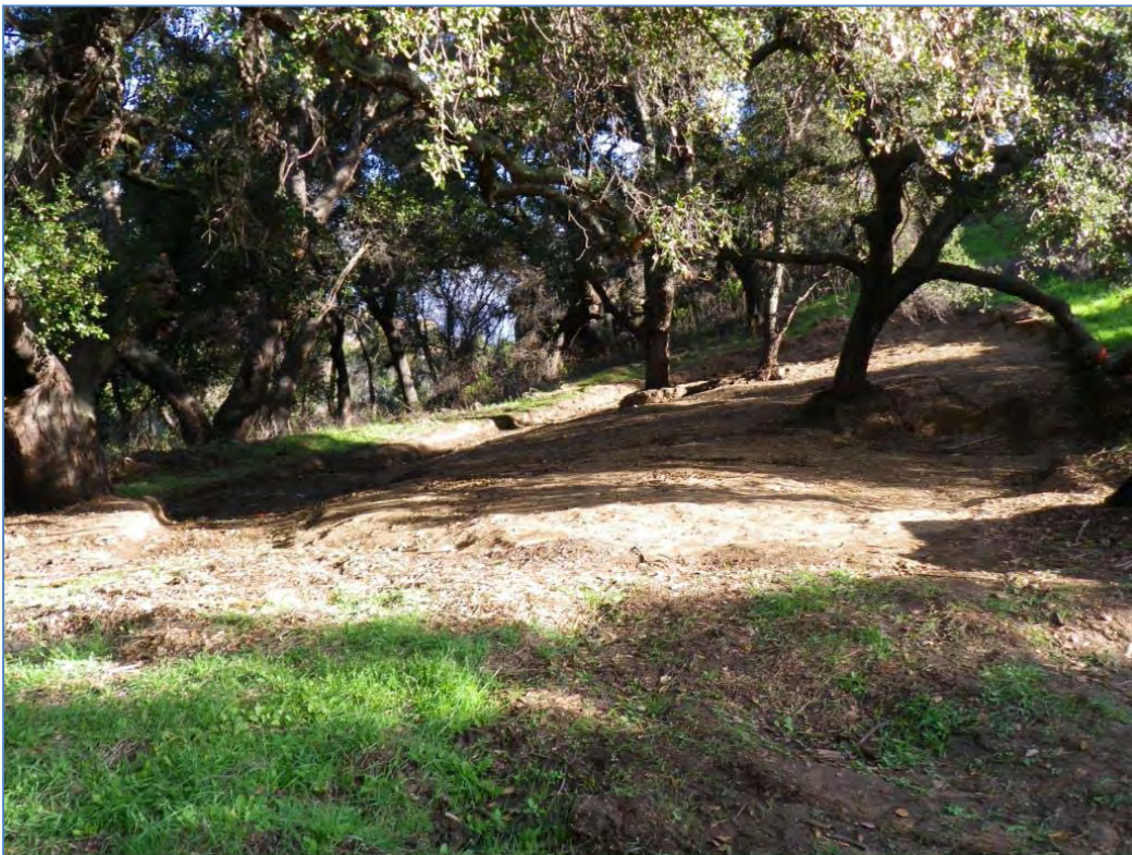
ISRA area AP/STP-1F after excavation (11/23/2010, looking northeast).
