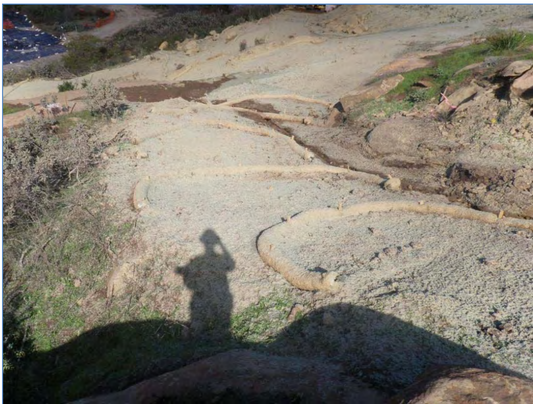
ISRA area B1-1C in foreground and B1-1B in background after restoration (11/23/2010, looking north). Faded blue-green hydroseed mulch is visible.
