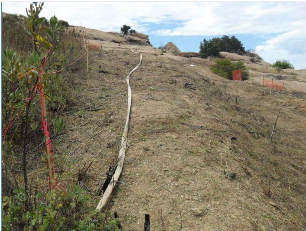
ISRA area B1-1B, after vegetation clearance, prior to excavation (7/16/2010, looking south). Orange fencing around Santa Susana tar plants.
