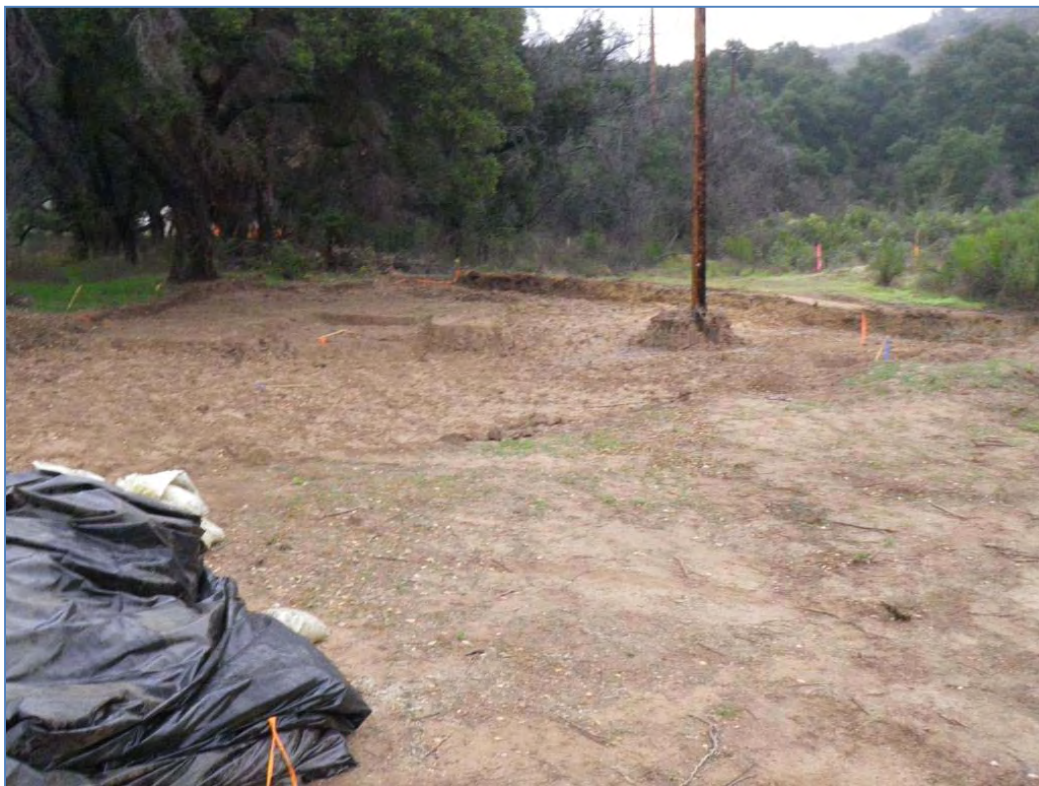
ISRA area AP/STP-1D after excavation (11/19/2010, looking east).
