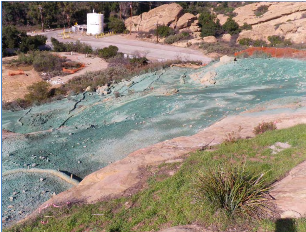
ISRA area B1-1B after restoration (11/16/2010, looking north). Blue-green hydroseed mulch is visible.
