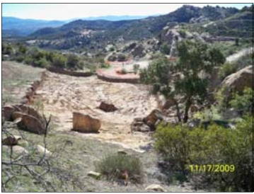
HVS-2A Completed excavation (looking South). November 2009
