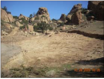
HVS-2A Completed excavation (looking North). October 2009
