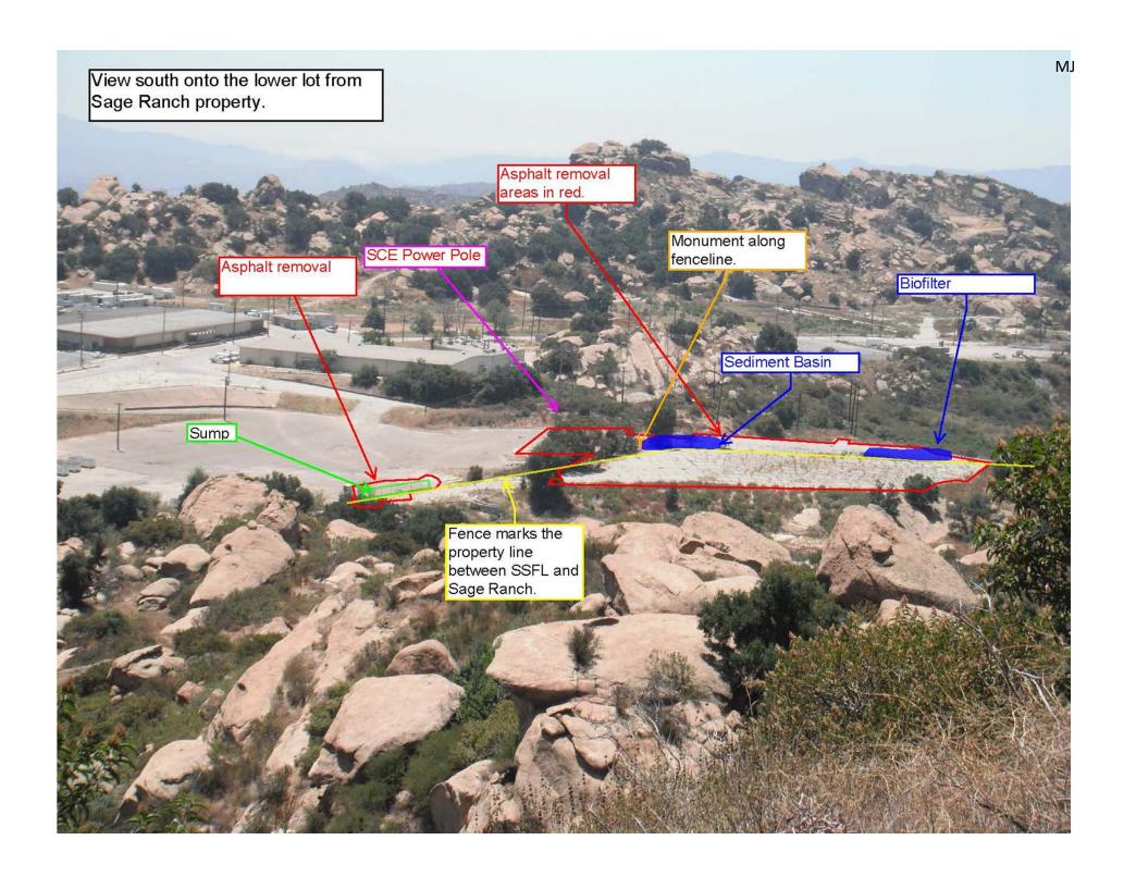
MJ **B1** Sediment Basin FRENCH DRAIN DISCHARGE PIPE REALIGN HOPE IO-INCH PIPE TO DISCHARGE DETAIL 5 ALONG THIS ROUTE SEE DETAIL 4 9 EXISTING DRAINAGE HOPE 10-INCH PIPE. SEE NOTE ! DETAIL 3 • SEE NOTE 4 1 FRENCH DRAIN TO BE INSTALLED. SEE NOTE 2 Treat runoff from ~2 acres including **RFI & ISRA areas** Design complete, construction planned to begin soon
