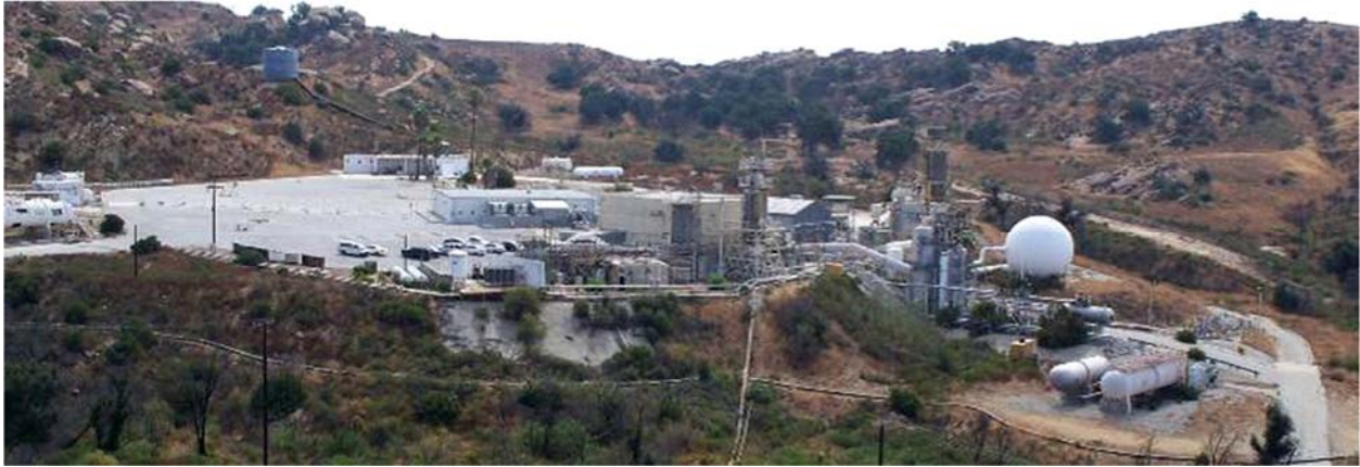
Figure 5: CTL3 – Original Buildings/Structures
