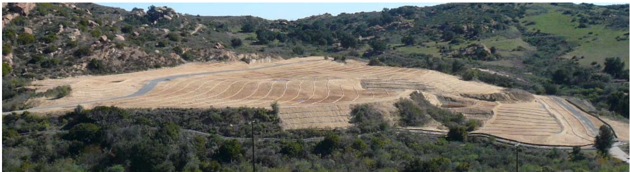
Figure 6: CTL3 – Stabilization after Demolition
