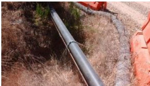
Picture #14: Looking south at HDPE pipe crossing culvert.
