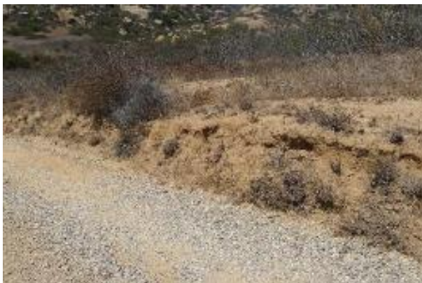
Picture #20: Looking west at escarpment on north side of road.
