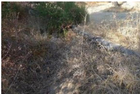
Picture #5: Looking southwest at erosion underneath HDPE pipe.
