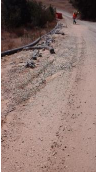
Picture #16: Looking south at old fiber roll check dams and rip rap.
