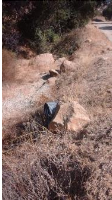
Picture #11: Looking north at gravel in drainage and culvert pipe.
