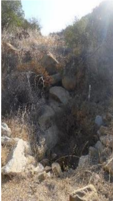
Picture #10: Looking east at rocky hillside upslope of erosion.
