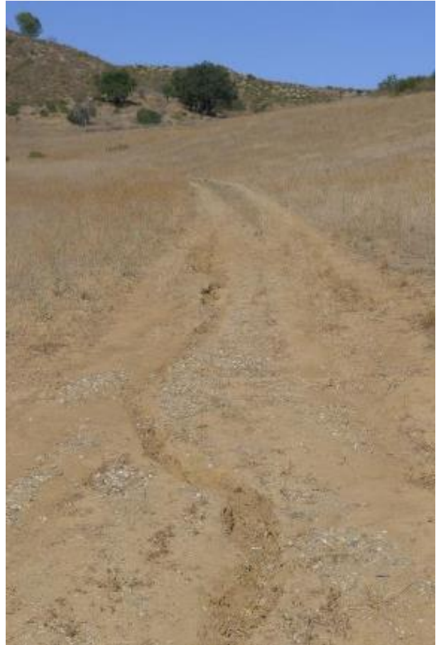
Picture #36: Looking east at rill development across road.
