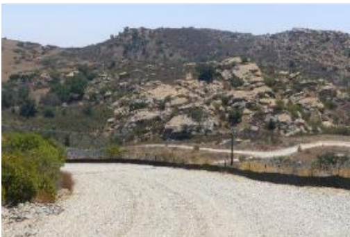
Picture #18: Looking south at silt fence and gravel water bar.
