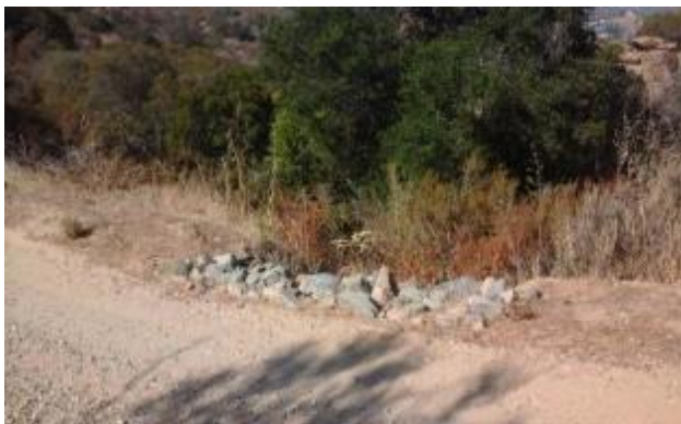
Picture #7: Looking southwest at rip rap placed at discharge point.
