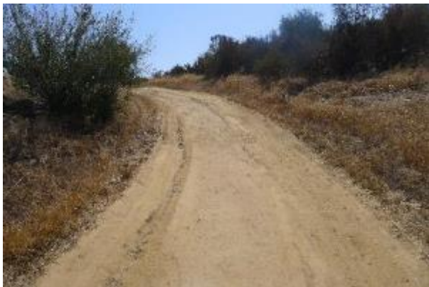
Picture #13: Looking east at minor erosion on road surface.
