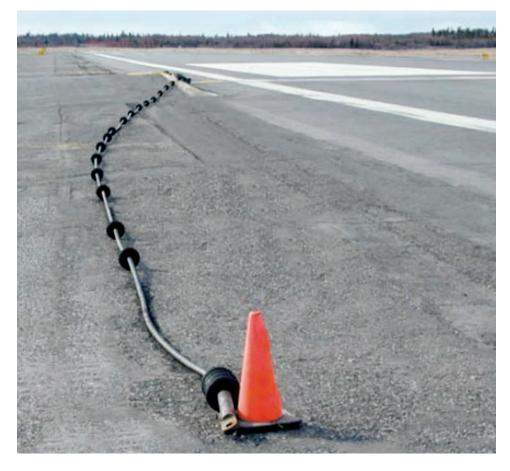
At the majority of joint-use airports in the United States, this modification has been made to the standard BAK-9/-12/-13 systems that previously were supported by rubber donuts. Worldwide, there are approximately 500 BAK-14 and 25 Type H systems installed. Roughly 95 percent of joint-use runways have BAK-14 or Type H modifications installed. (See the definition of *BAK* in "Common terms" on page 20.)
