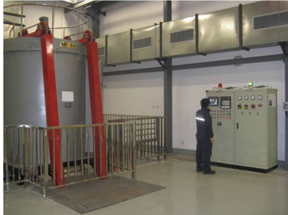
Heat treatment shop
